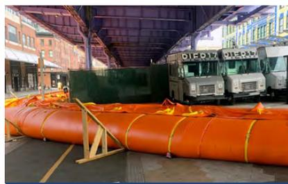
Water-filled Tube Barrier
